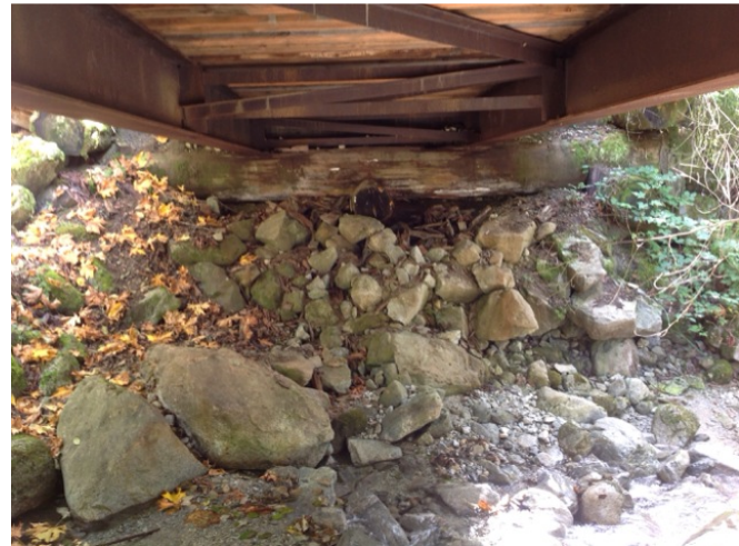
Left Bank Abutment when facing downstream
