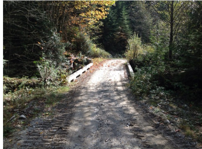
Approach from Right Bank when facing downstream
