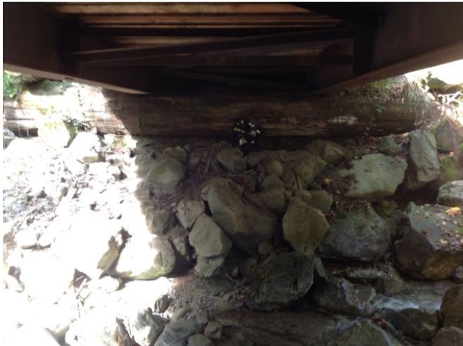
Right Bank Abutment when facing downstream
